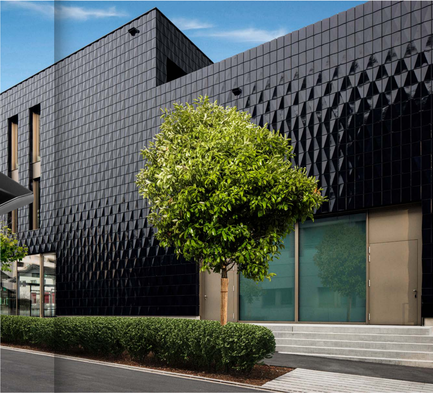
DREIKLANG A and B (diagonal line to the left or right) Dimensions: 14,5x9x2 cm Tiles per m 2 : 64
